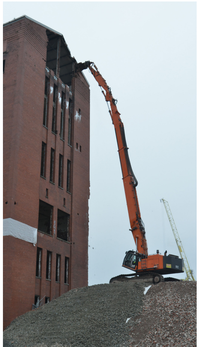
Figure 9: A high reach demolition machine using a ramp as protection from debris and to gain reach
