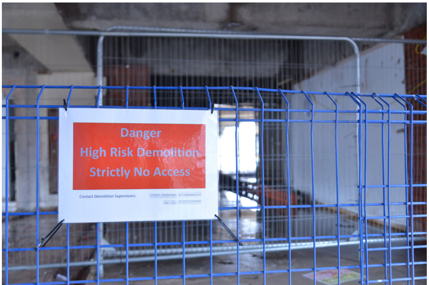
Figure 1: Fencing for an AMBER ZONE
