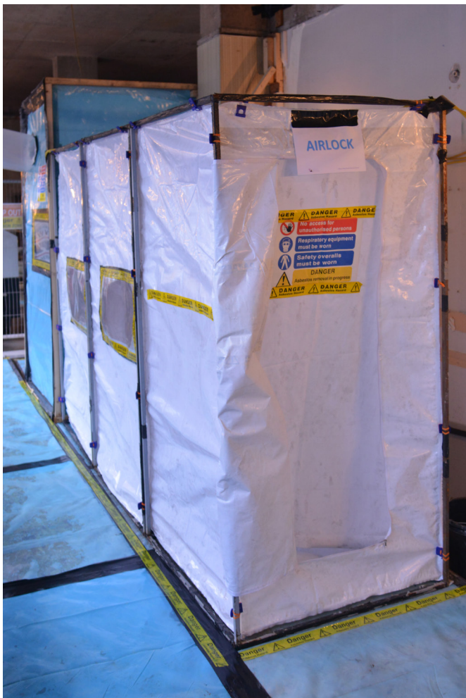
Figure 4: Licensed asbestos removal work has its own specific standards for creating AMBER exclusion zones – signage on a 3-stage airlock
